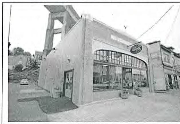
Figure 14.115-5: Non-Industrial Building, Flat Roof Behind Parapet Wall
