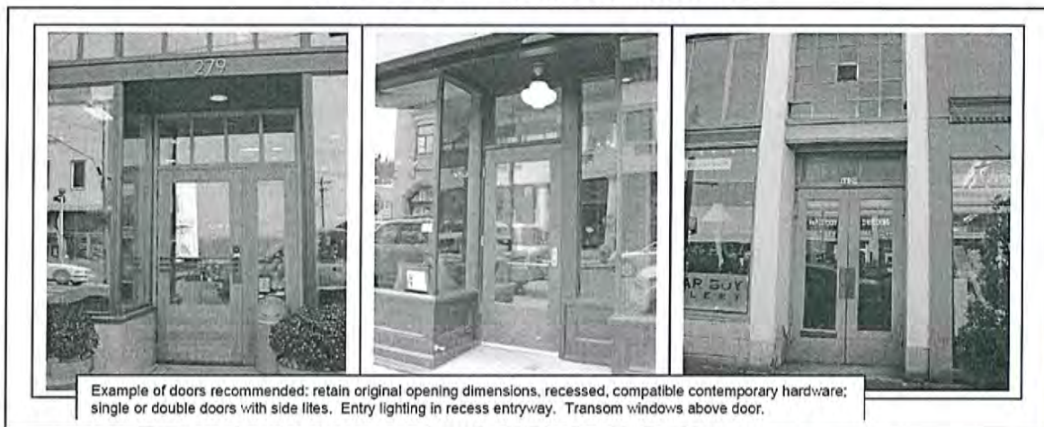
Figure 14.115-9: Recessed Doors, Contemporary Door Hardware, Single/Double Doors, Side Lites, and Transom Windows
