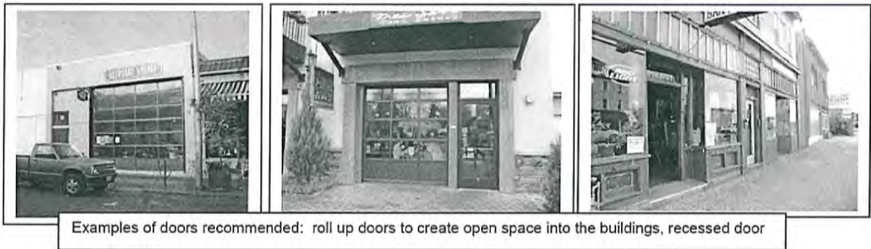
Figure 14.115-8: Roll-Up Doors and Recessed Doors
